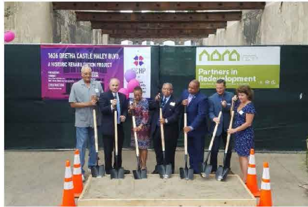
NORA and development partners join for a groundbreaking at the last vacant building in the 1600 block of Oretha Castle Haley Boulevard.
