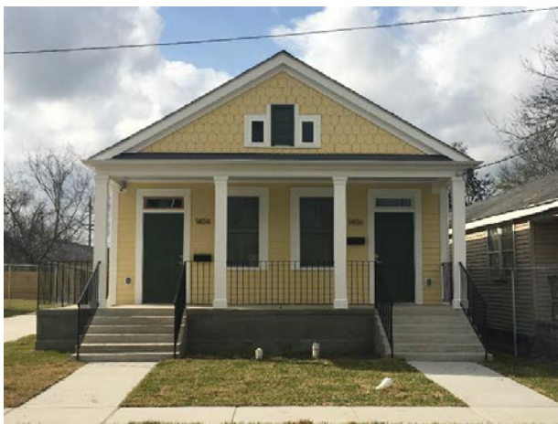
Blueberry Hill Homes property in Lower Ninth Ward
